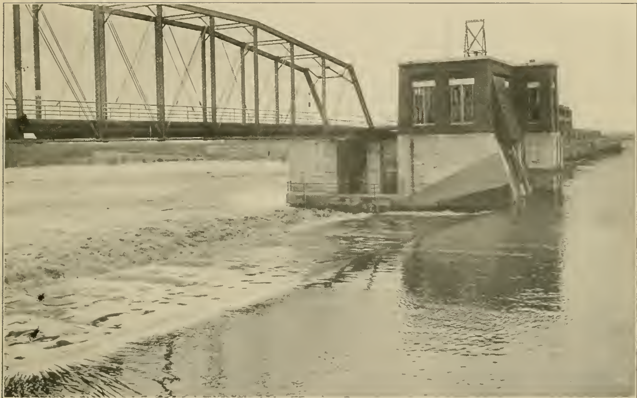
A VIEW OF THE CONTROLLING WORKS ON THE DRAINAGE CANAL. Bear trap dam at Lockport looking down stream.
