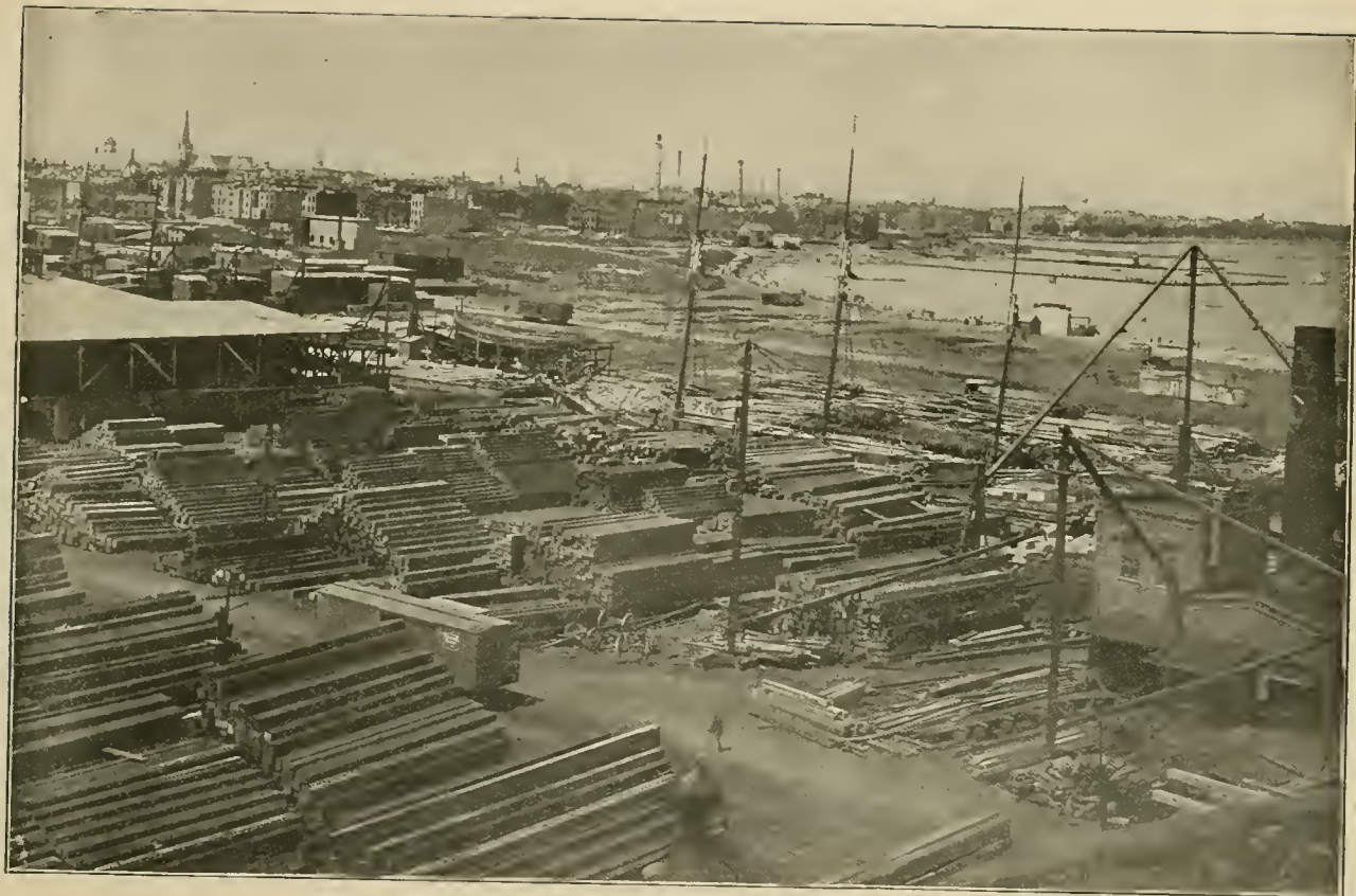
BIRD'S-EYE VIEW FROM THE NORTH PIER LIGHTHOUSE.
